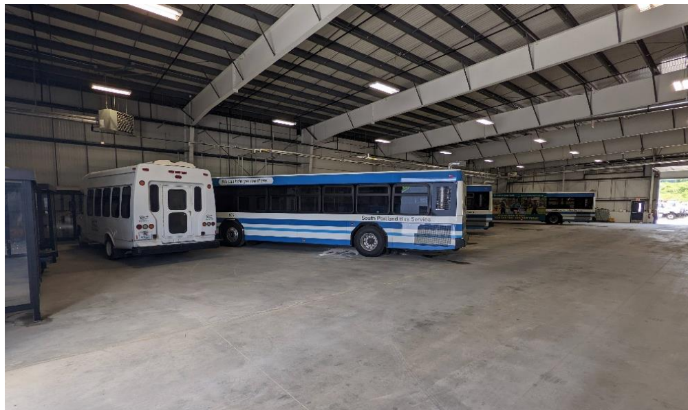
Figure 7 Bus Storage Bays
