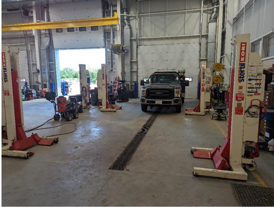
Figure 6 Main Vehicle Maintenance Area
